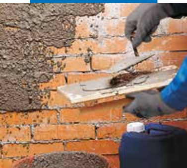
Base-keying mortar layer with Planicrete admix
