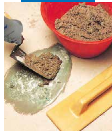
Floor patching: application of mortar
