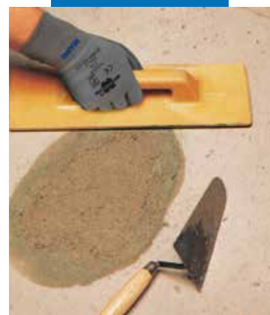
Floor patching: final smoothing
