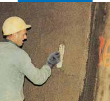
Cement plaster with Planicrete - Ville Marie motorway tunnel, Montreal, Canada
